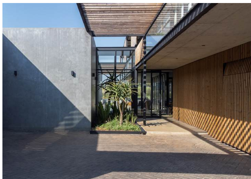
The garage door, featured with Lunawood battens, is camouflaged in the wall.
